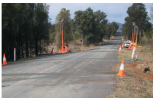
Repair works to Charlton Road.
