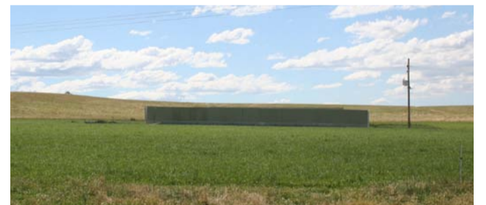
Noise and visual screening of a gas well on private property near Charlton Road.
