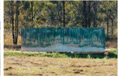
Painted Colorbond walls
