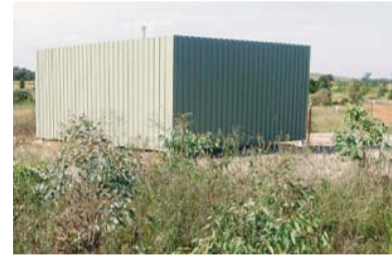
Colorbond walls shielding gas well
